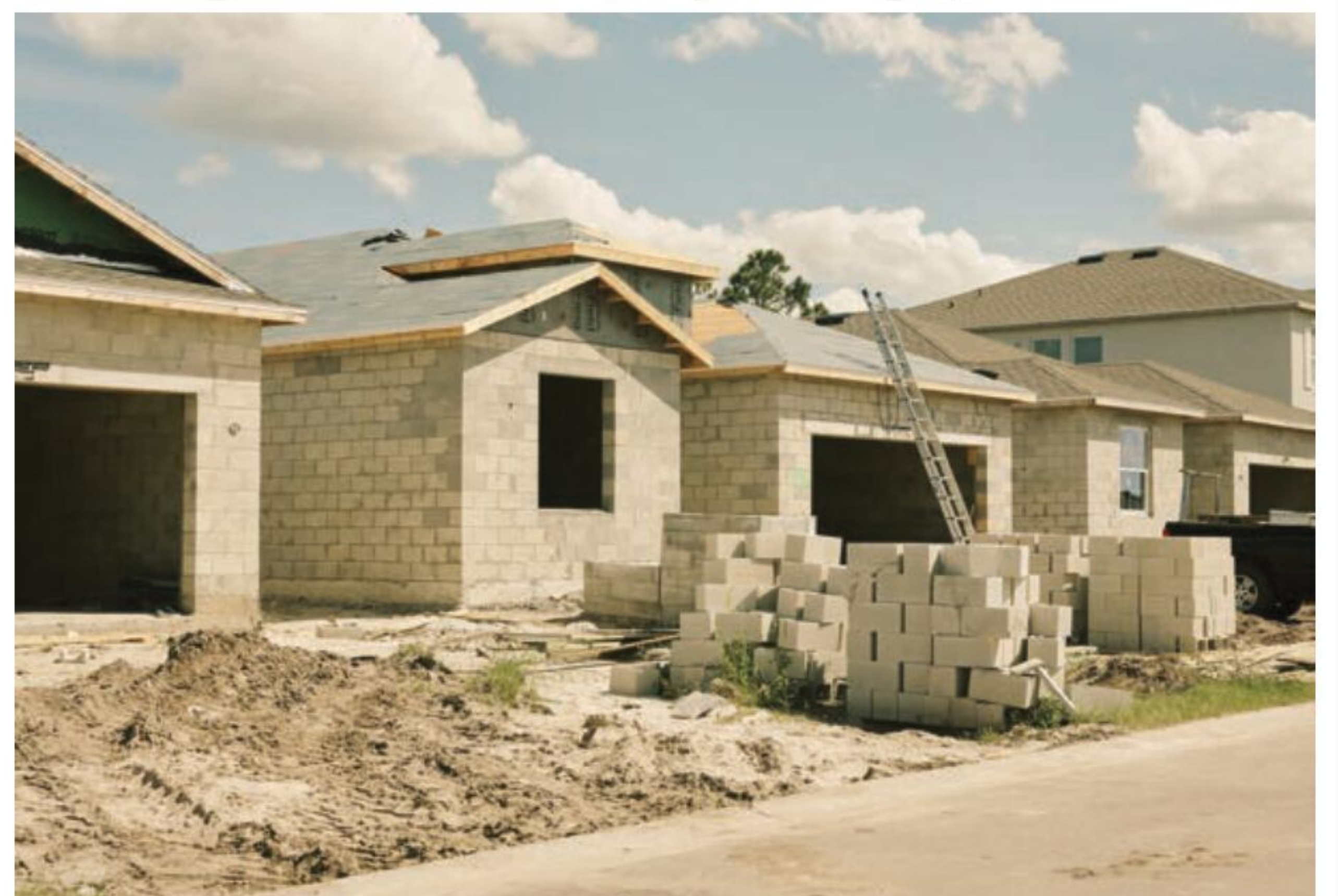
▲ Homes under construction in Lakewood Ranch, Fla.
